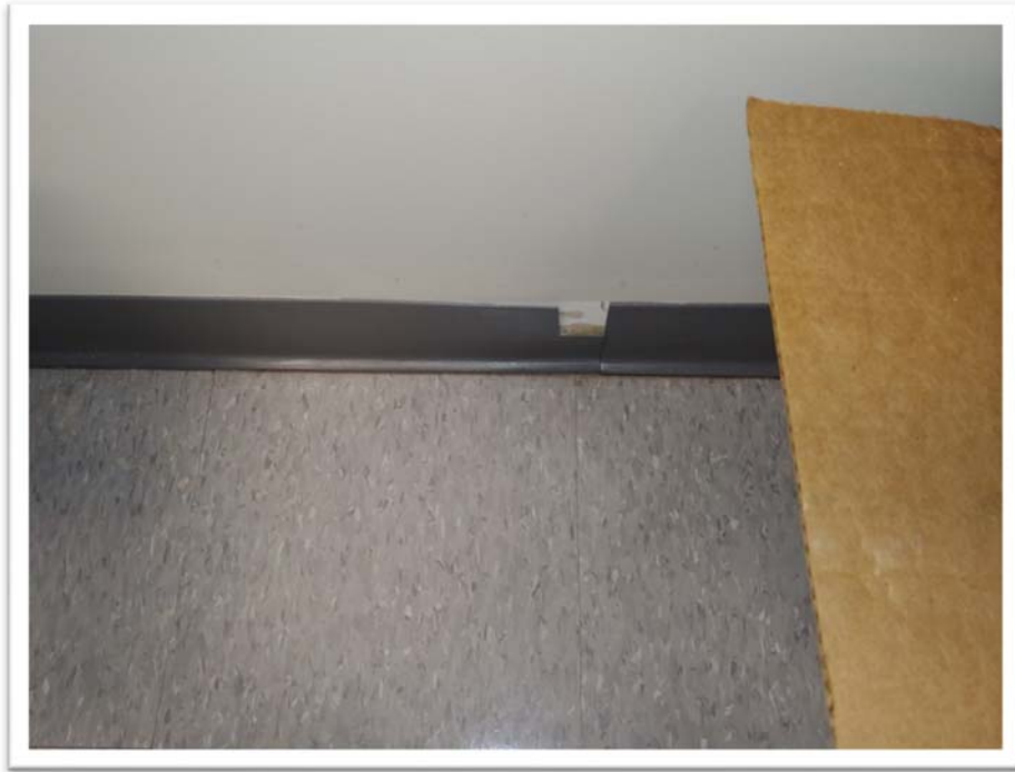
Photograph #013 View of the dark gray cove base sampling point (None Detected).
