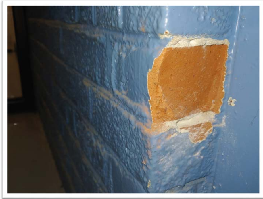
Photograph #015 View of brick and grout sampling point (None Detected).
