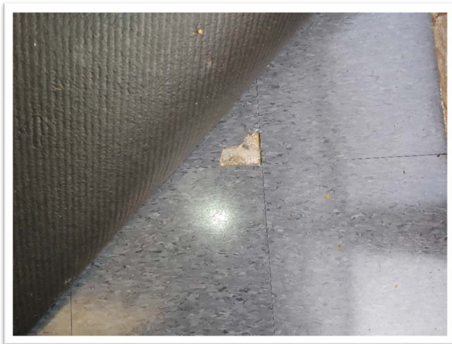
Photograph #012 View of dark gray vinyl floor tile/mastic sampling point VF-6 (None Detected).
