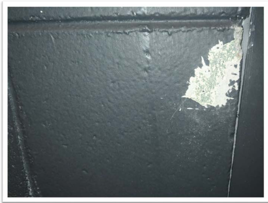
Photograph #016 View of CMU block filler surface coating sampling point (None Detected).
