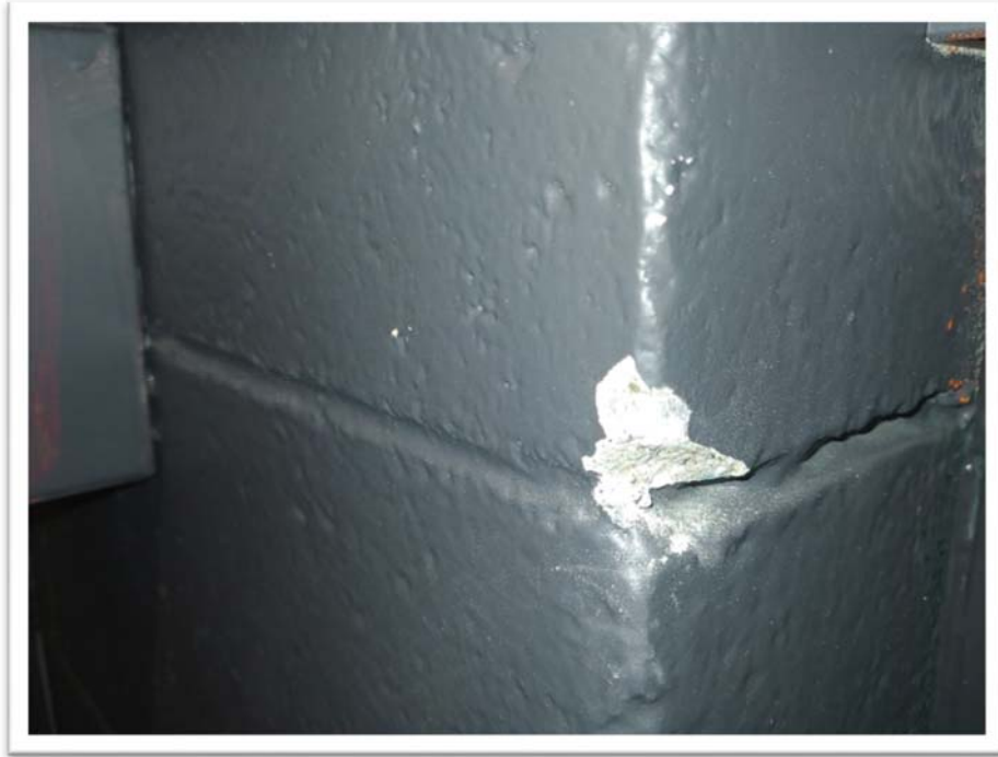
Photograph #017 View CMU block and mortar sampling point (None Detected).
