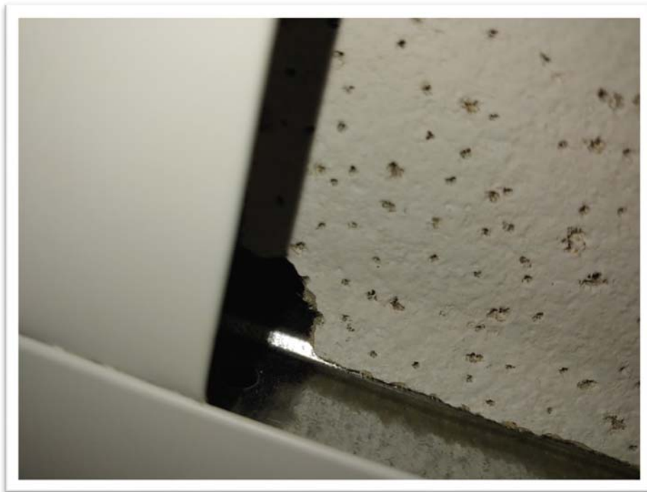
Photograph #014 View of ceiling tile sampling point (None Detected).
